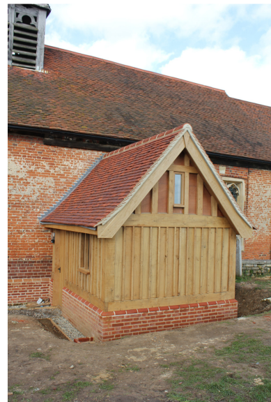
New Toilet Extension
