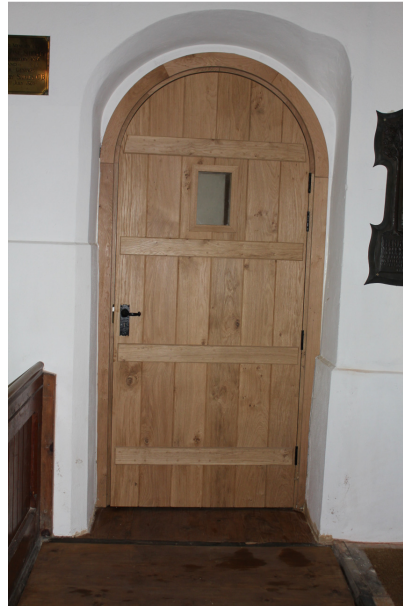
Re-opened South Door
