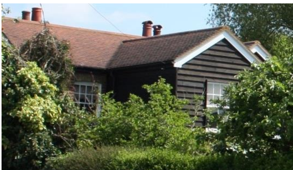
Fig. 5 Black painted weatherboarding at Ferndale
