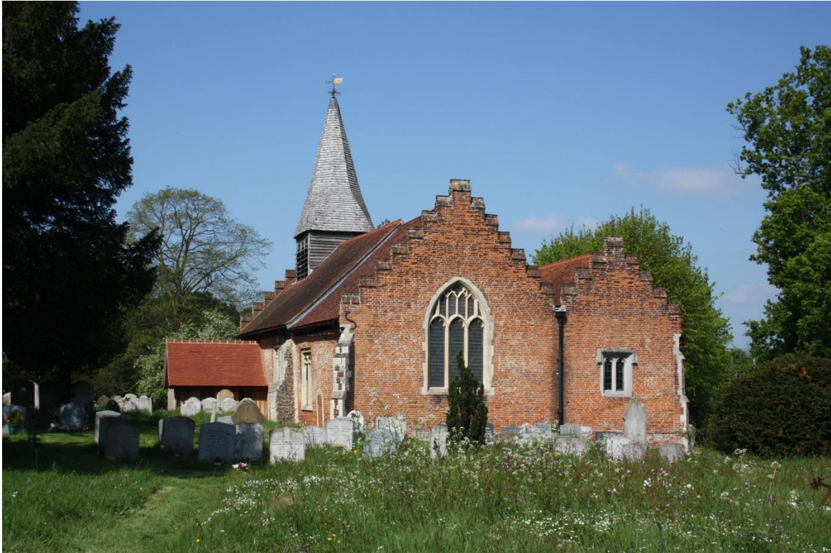
Fig. 33 The parish church view from the east
