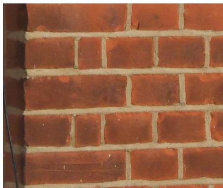
Fig. 8 Brickwork on the almshouses (1908)
