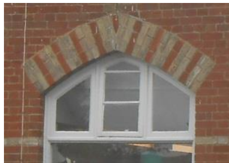
Fig. 7 Brickwork on the primary school (1873)
