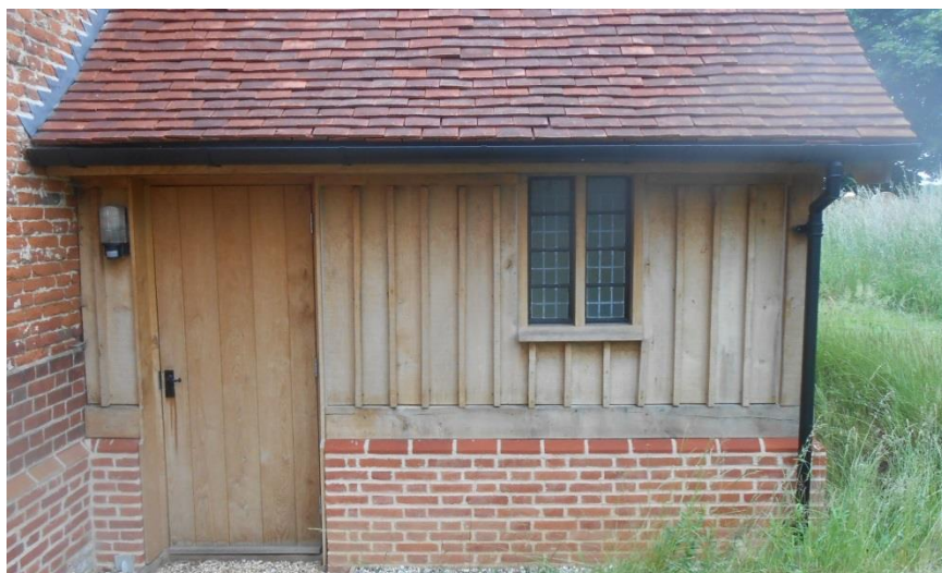
Fig. 3 Un-painted oak cladding on the recent extension to the parish church
