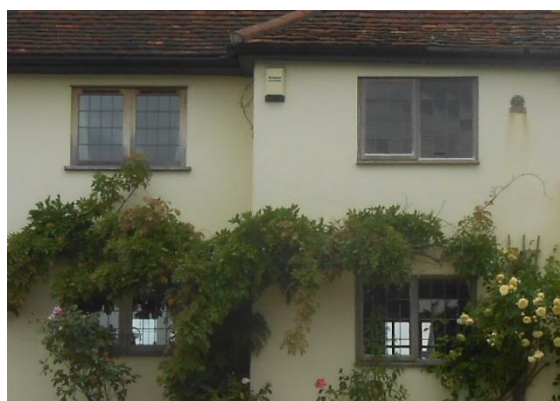
Fig. 17 Lead-glazed windows in unpainted oak frames
