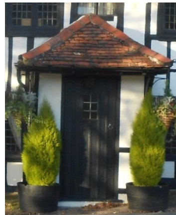
Fig. 23 Timber door with vertical batten stained black
