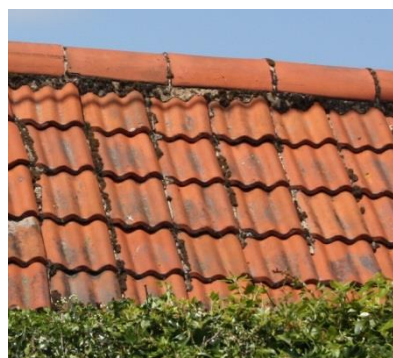
Fig. 11 Single-lap clay pantiles
