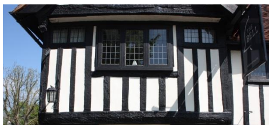
Fig. 2 Exposed timber framing on The Bell
