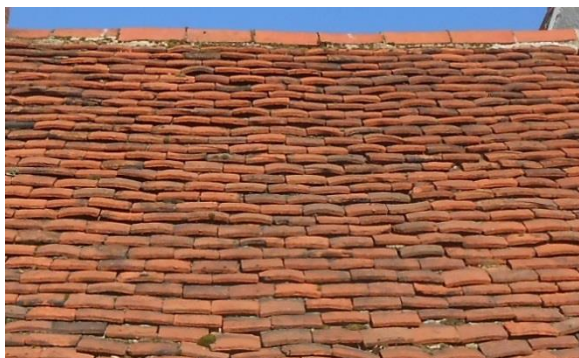
Fig. 10 Double-cambered clay plain tiles
