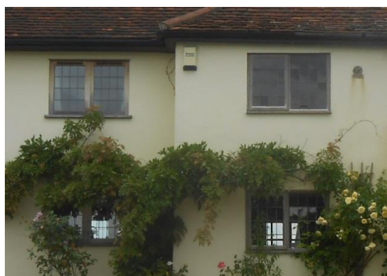
Fig. 17 Lead-glazed windows in unpainted oak frames
