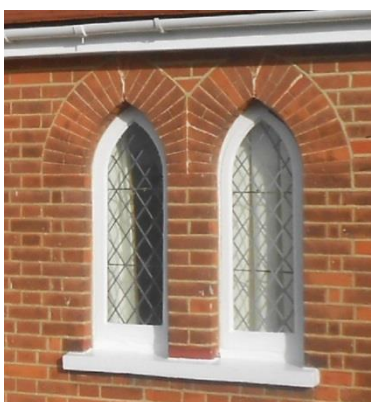
Fig. 16 Early 20 th -century lead-glazed windows with pointed arch heads
