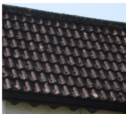
Fig. 13 20 th -century concrete tiles
