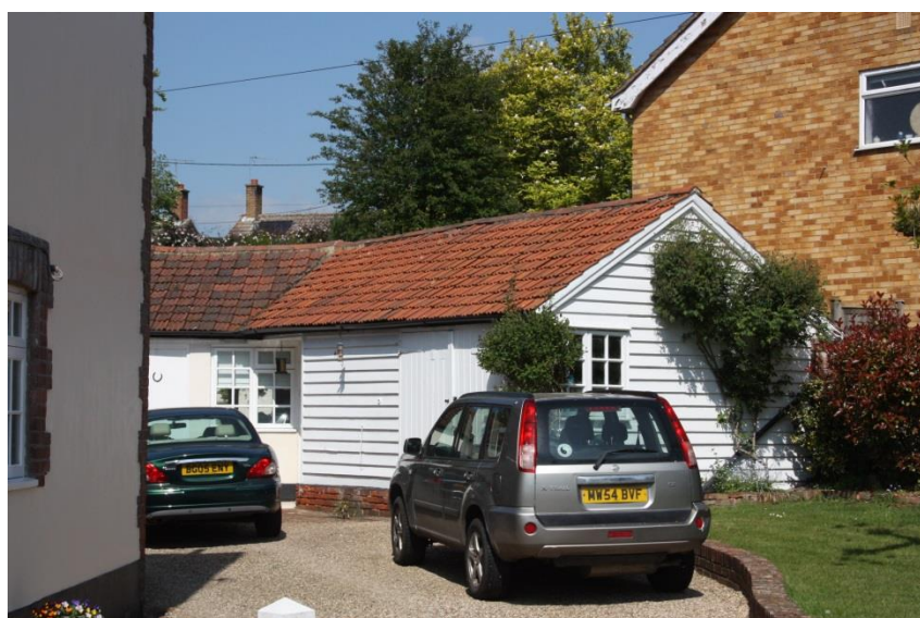
Fig. 4 White painted weatherboarding at Lynton
