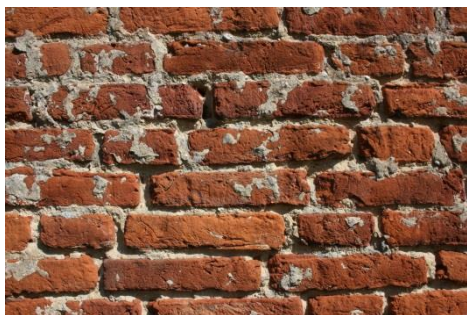
Fig. 6 Brickwork on the parish church (1562-4)
