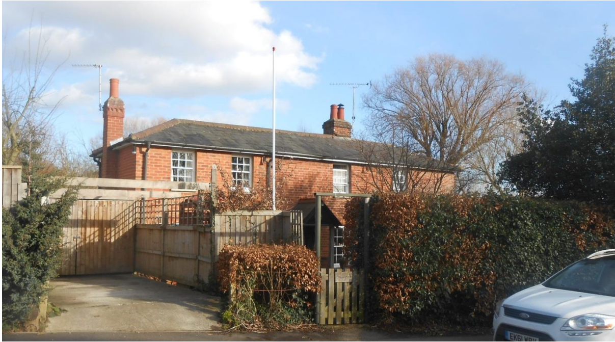
Fig. 52 2 Brick Cottages (left) and 1 Brick Cottages (right)
