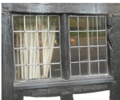
Fig. 14 Early 17 th -century mullion window
