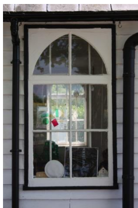
Fig. 18 Arch headed casement window
