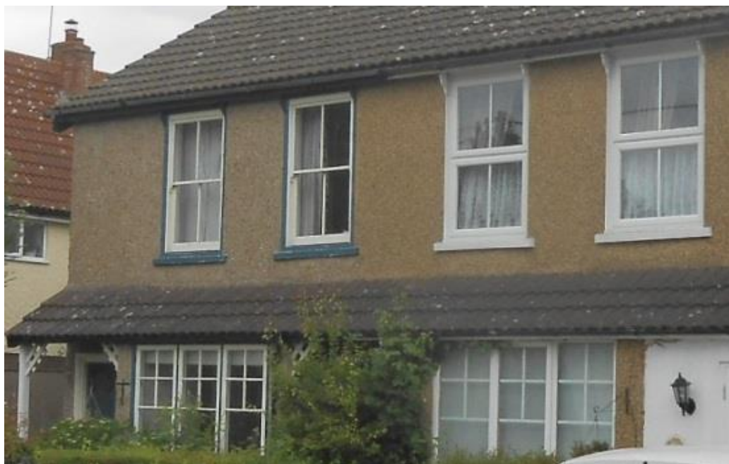
Fig. 20 Original painted timber windows and plastic replacement windows
