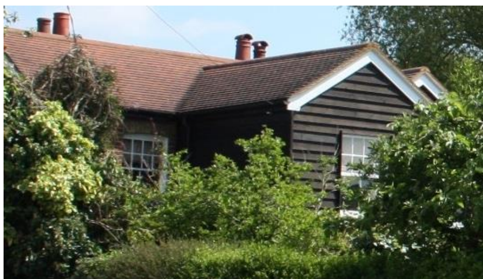
Fig. 5 Black painted weatherboarding at Ferndale
