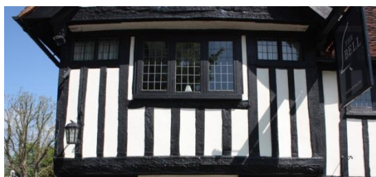
Fig. 2 Exposed timber framing on The Bell
